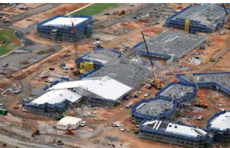
Aerial view of the new South Queensland Correctional Precinct.
